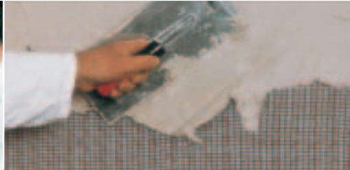
Simply lay on plaster with a trowel.
